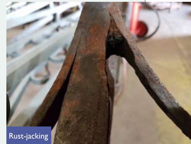
Blistering, pitting and rust-jacking
