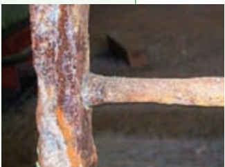
Top: Wrought iron stile and rail: - 1858 - material sections still intact
